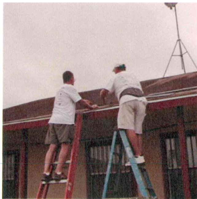
Replacing rotten wood Joel's office by Azle Mission work group 2017.
